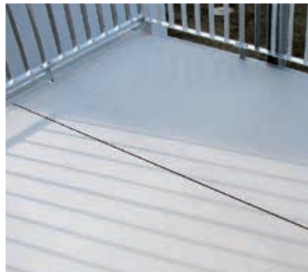
INCLINE AND PANEL JOINTS
