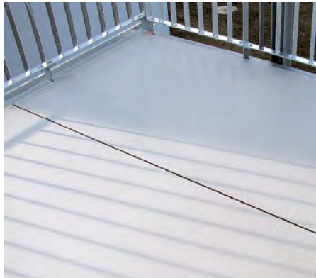
INCLINE AND PANEL JOINTS
