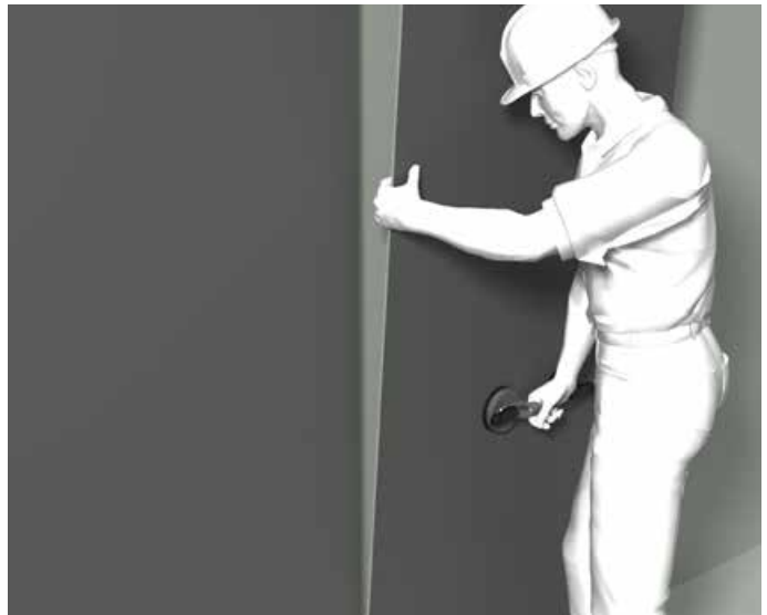
Place panels with suction handles
