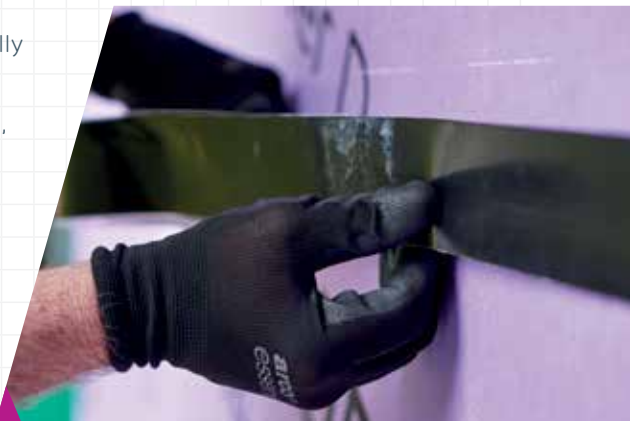
weather defence™ Joint Tape being applied
