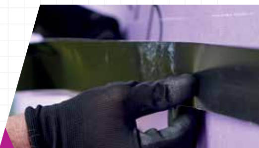
weather defence™ Joint Tape being applied
