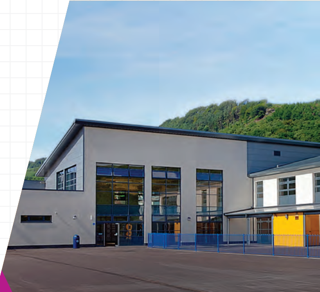
Abercynon Primary School, South Wales
