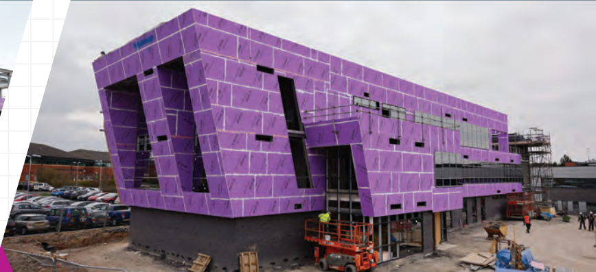
Wales & West Housing Office, Deeside
