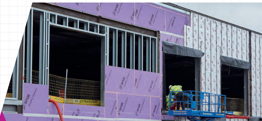
Insulation on Weather Defence
