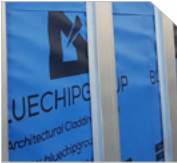
ULTRAPERM Class 4 Membrane
